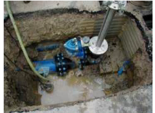
Inserting into hydrant fitting
